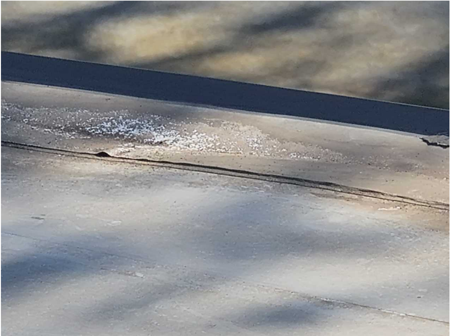
103 98-Loose Seams Date Taken: 4/21/2025 Taken By: Angela Night Edges around the roof membrane are separating from their seams due to poor installation and gap movement.
