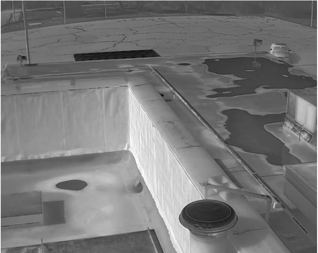
77 77-Loose Seams Date Taken: 4/21/2025 Taken By: Angela Night Edges around the roof membrane are separating from their seams due to poor installation and gap movement.
