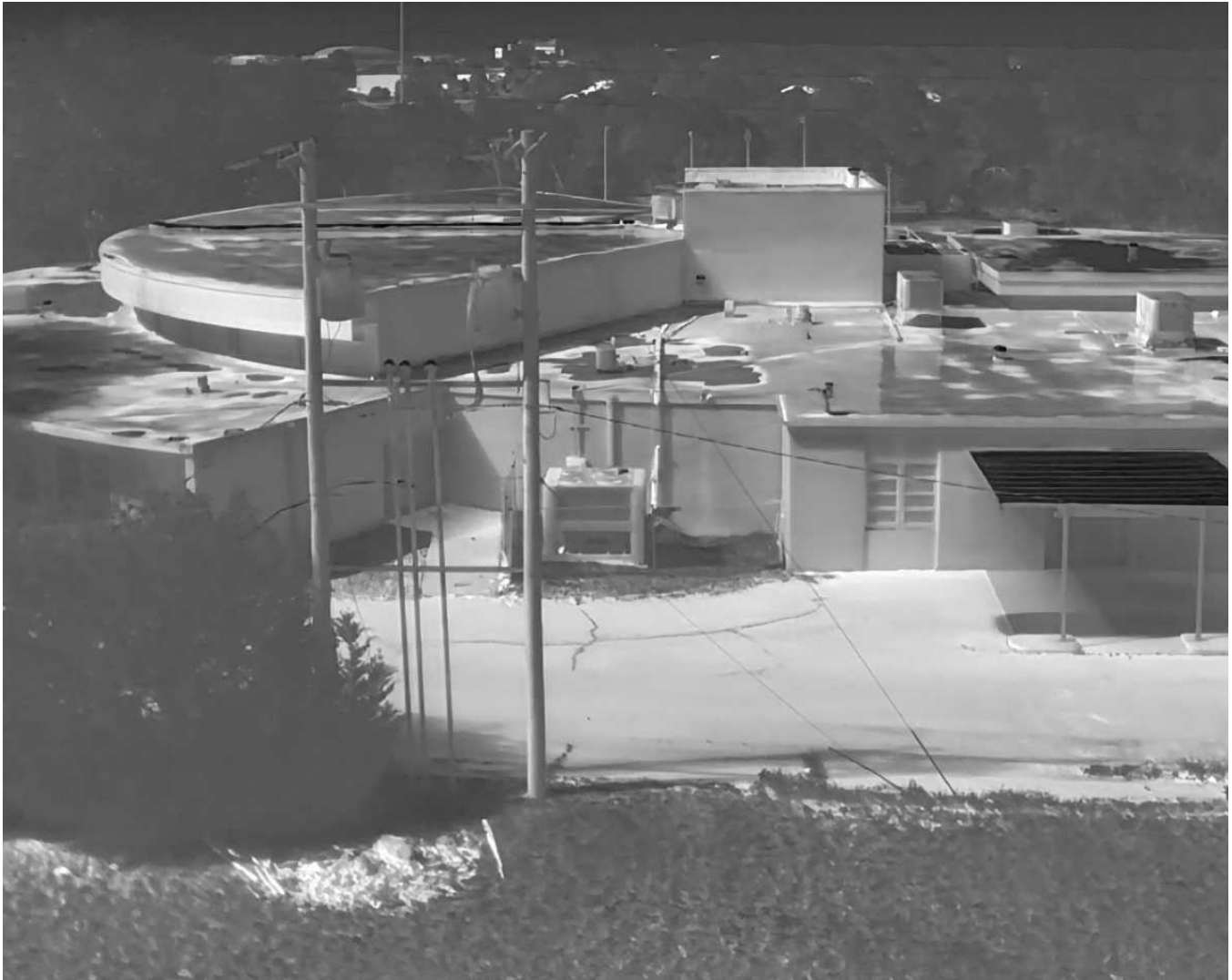
6 6-Ponding Date Taken: 4/21/2025 Taken By: Angela Night IR photos were taken in this instance to reflect the ponding of water due to leveling issues.
