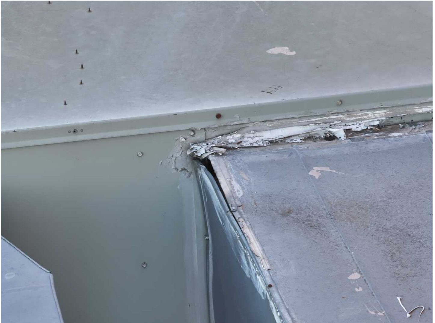
79 110-HVAC (Rectangular Duct) Date Taken: 4/21/2025 Taken By: Angela Night Exposed areas around the mechanical ducts were found atop the roof.
