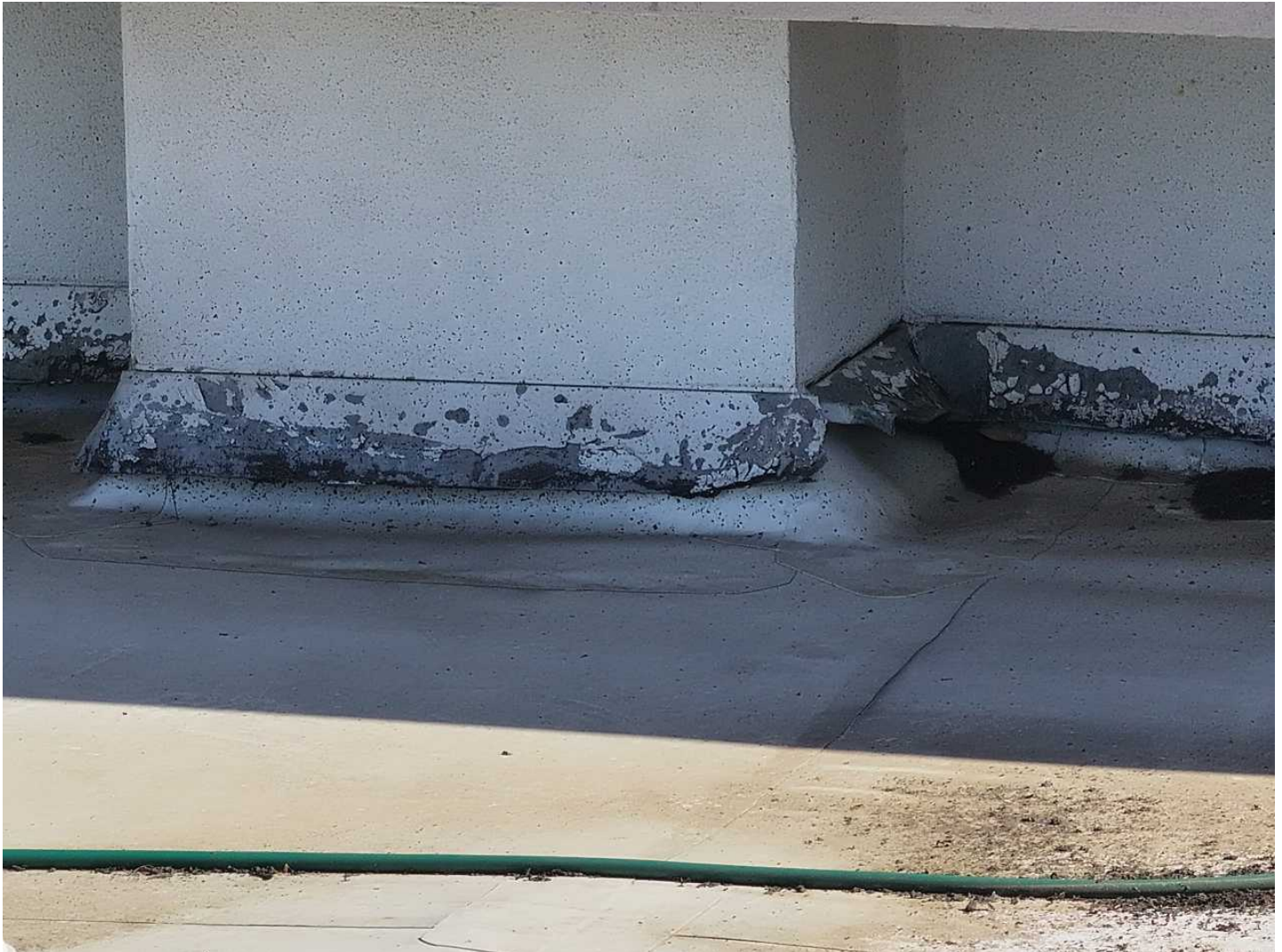
121 121-Failed Flashing Date Taken: 4/21/2025 Taken By: Angela Night Inadequate craftsmanship and unorganized placement indicative of a poor repair job or uncertified contractor.
