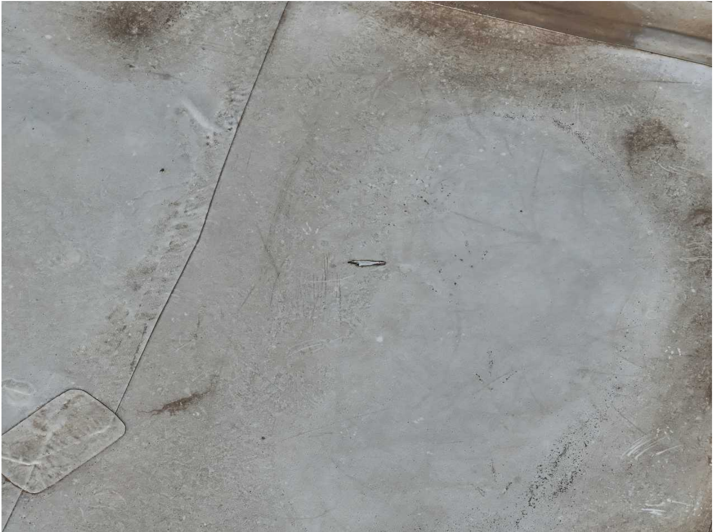
74 74-Mechanical Damage Date Taken: 4/21/2025 Taken By: Angela Night Splits are present on the roof that potentially were caused by irregular handling by roof repair companies.
