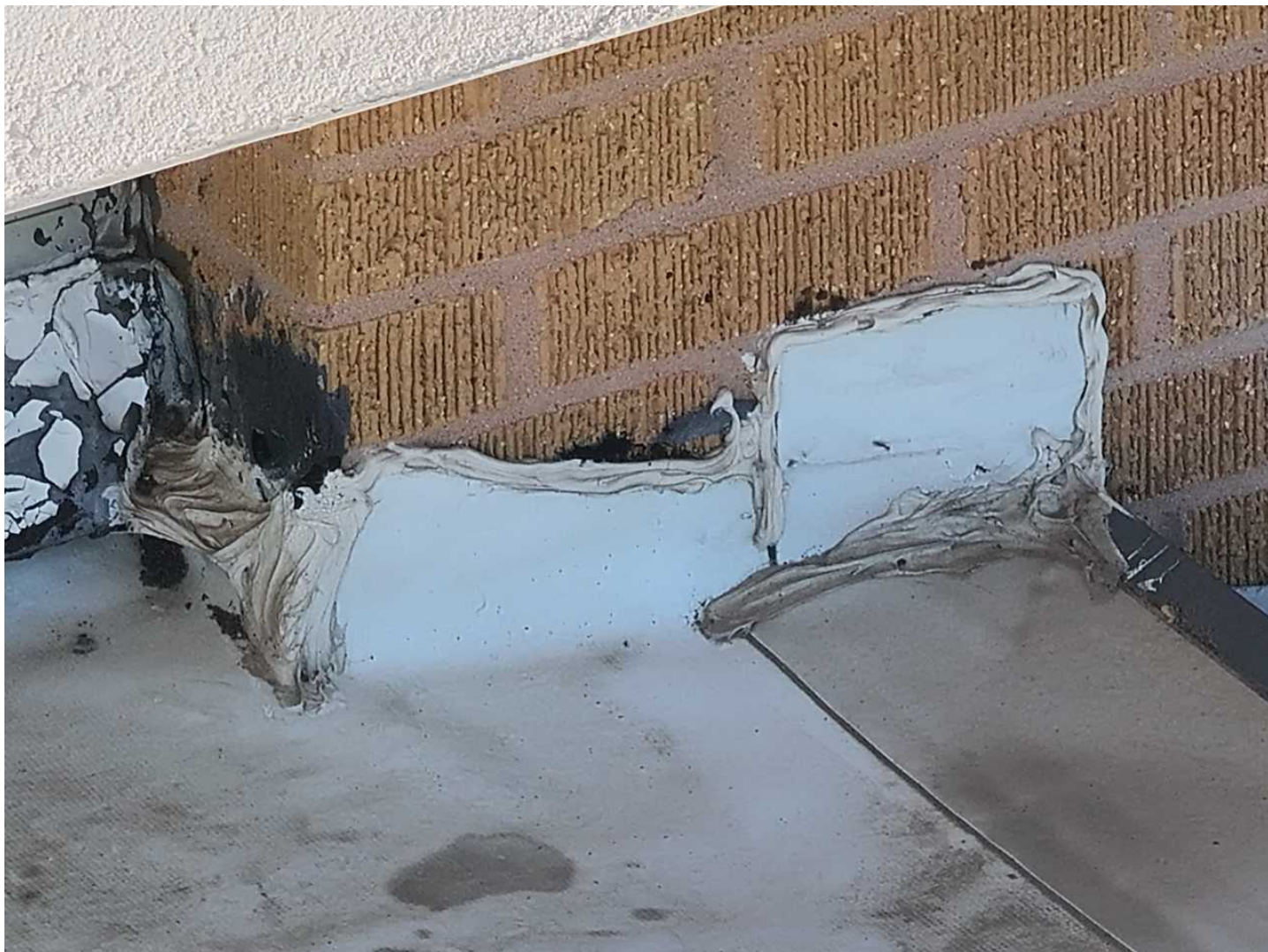
113 113-Failed Flashing Date Taken: 4/21/2025 Taken By: Angela Night Inadequate craftsmanship and unorganized placement indicative of a poor repair job or uncertified contractor.
