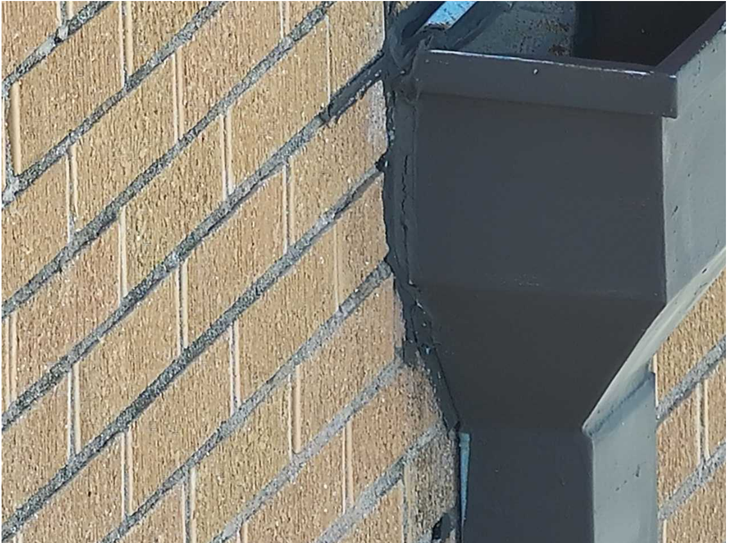
125 125-Conductor Head Need scrapped around and resealed
