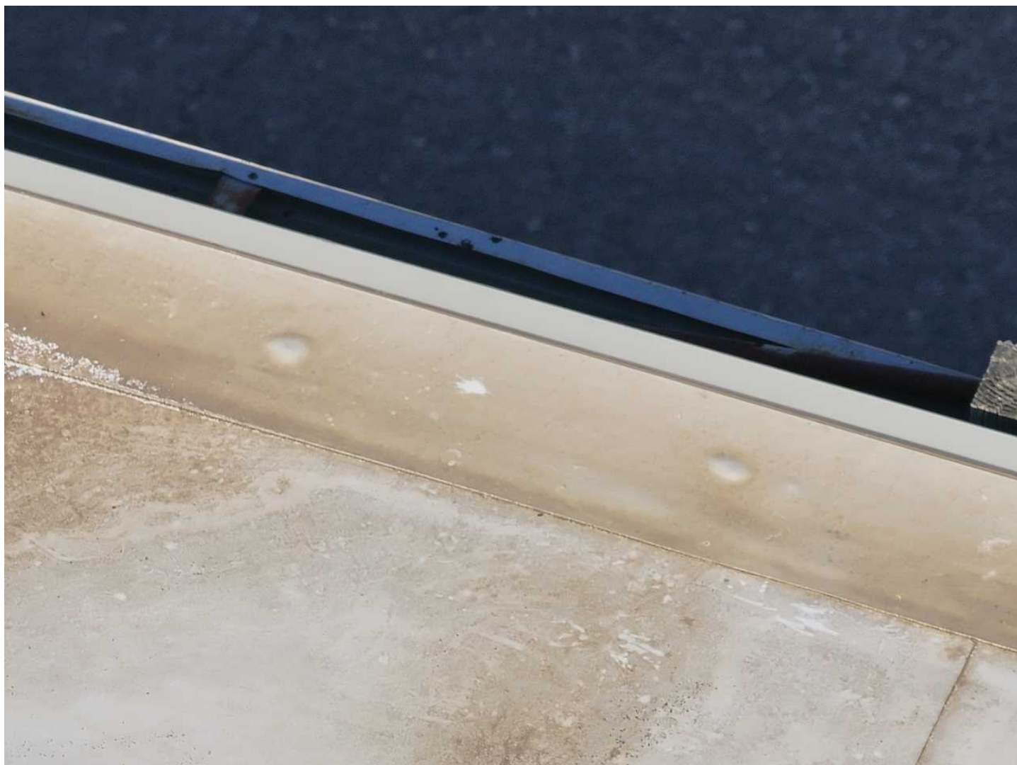
59 59-Indicative Hail Date Taken: 4/21/2025 Taken By: Angela Night Natural power wash markings from hail that was present (non damaging).
