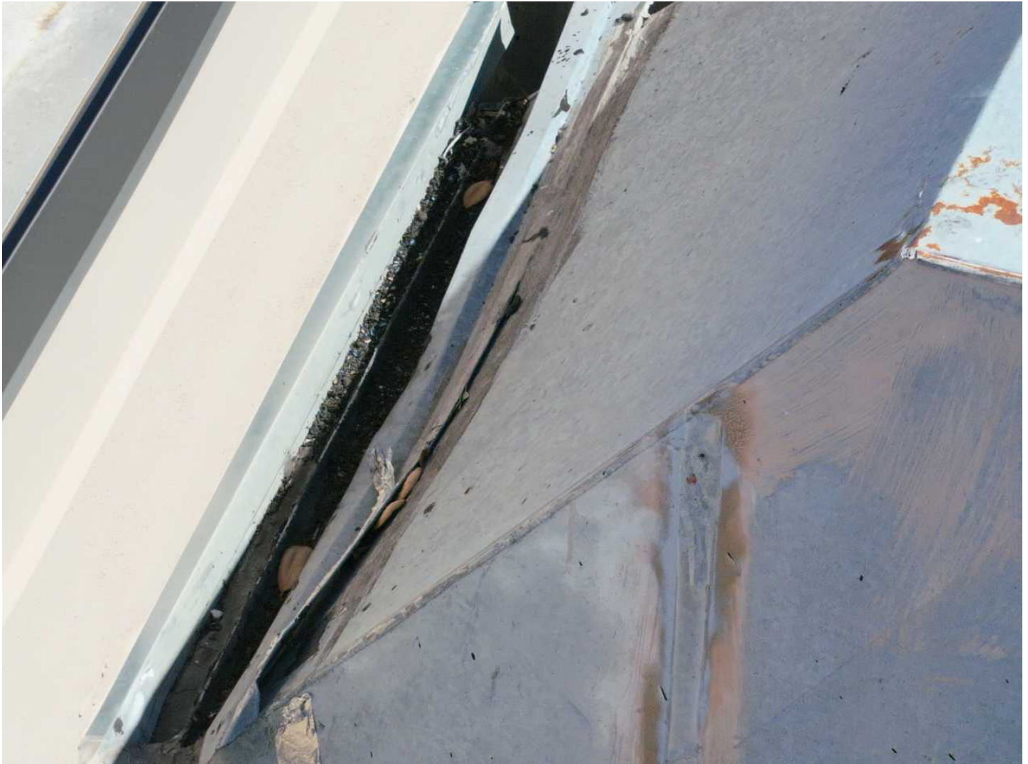
81 108-HVAC (Rectangular Duct) Date Taken: 4/21/2025 Taken By: Angela Night Exposed areas around the mechanical ducts were found atop the roof.
