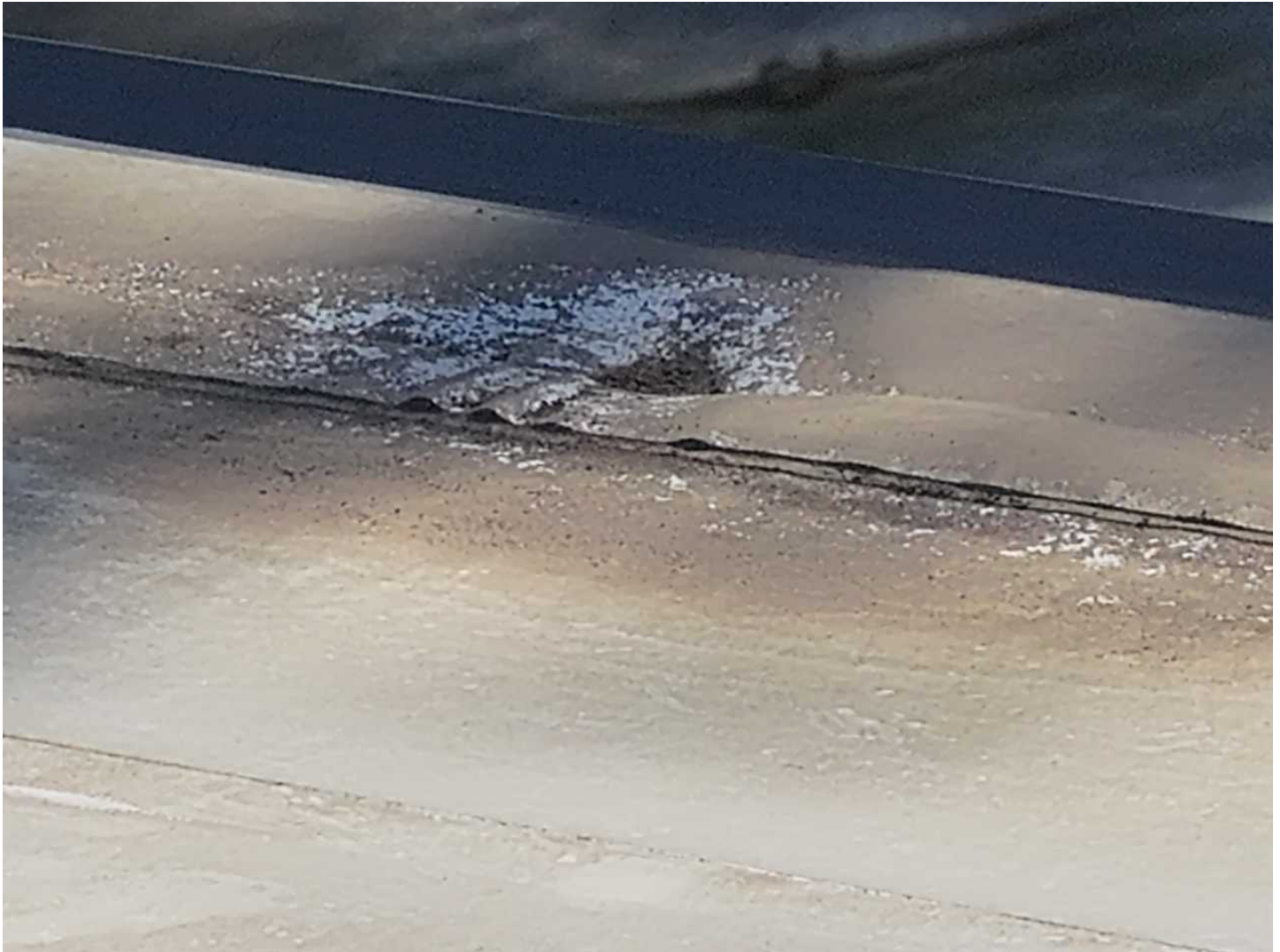
105 100-Loose Seams Date Taken: 4/21/2025 Taken By: Angela Night Edges around the roof membrane are separating from their seams due to poor installation and gap movement.
