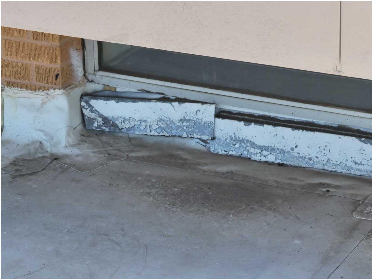
120 120-Failed Flashing Date Taken: 4/21/2025 Taken By: Angela Night Inadequate craftsmanship and unorganized placement indicative of a poor repair job or uncertified contractor.
