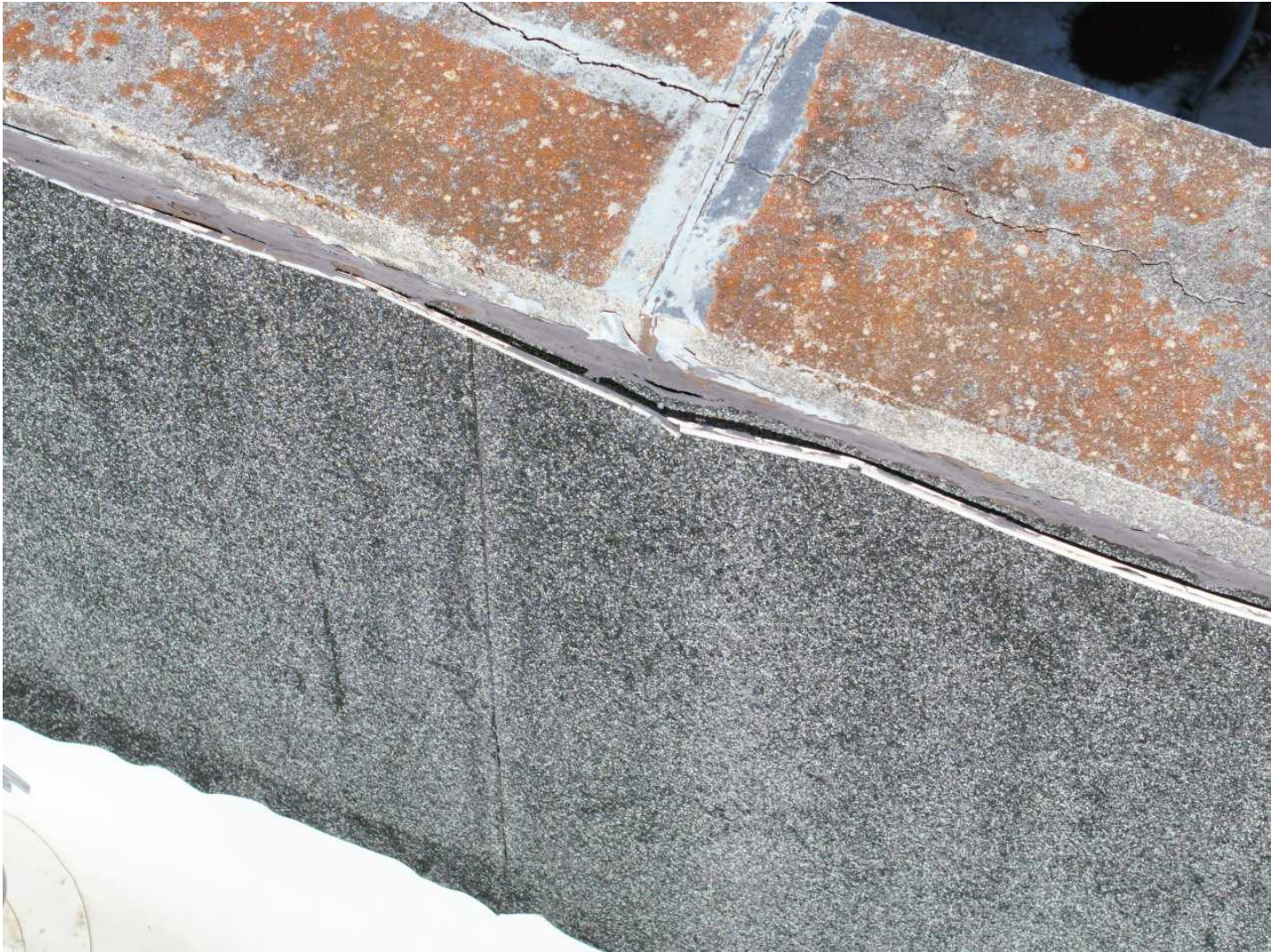
95 90-Loose Seams Date Taken: 4/21/2025 Taken By: Angela Night Edges around the roof membrane are separating from their seams due to poor installation and gap movement.
