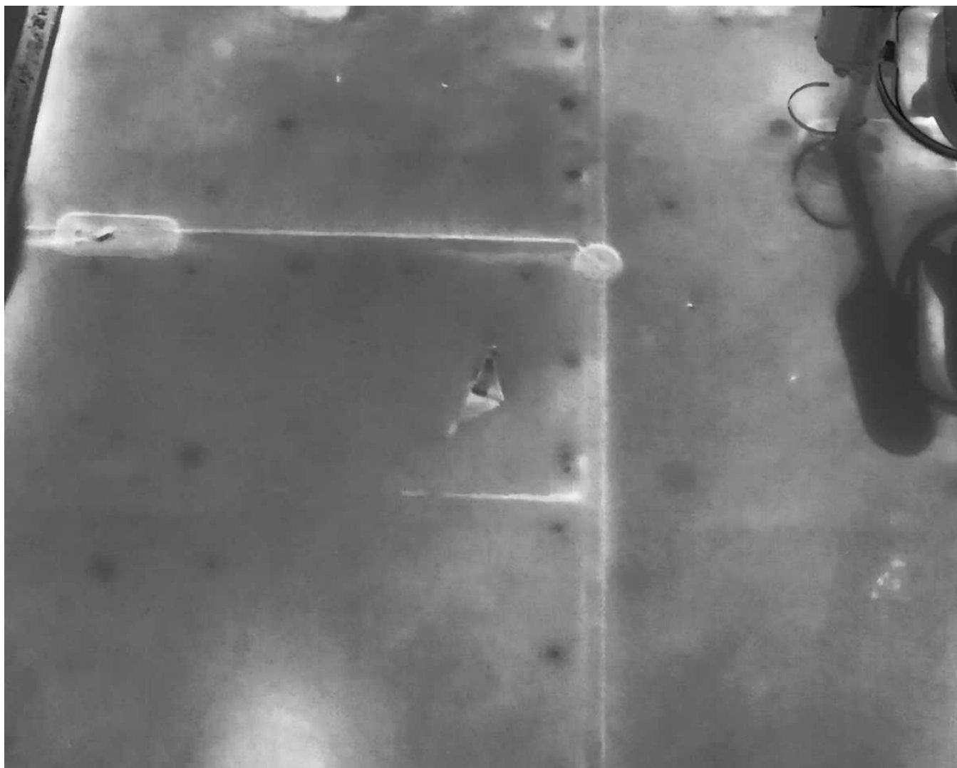
75 75-Mechanical Damage Date Taken: 4/21/2025 Taken By: Angela Night Splits are present on the roof that potentially were caused by irregular handling by roof repair companies.
