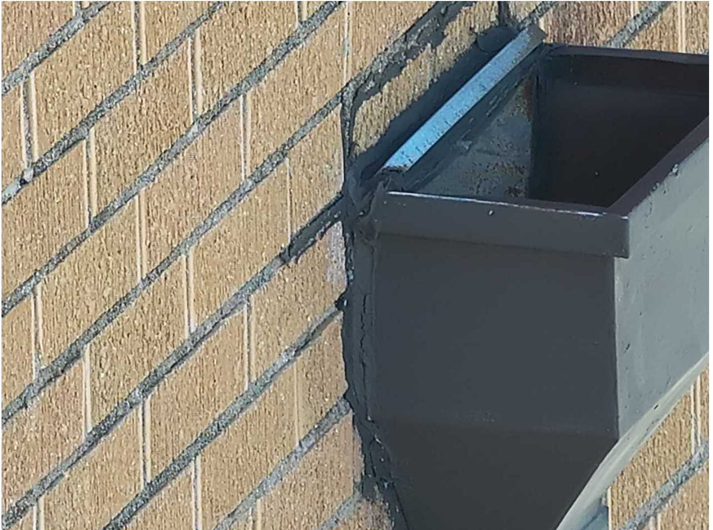
124 124-Conductor Head Need scrapped around and resealed
