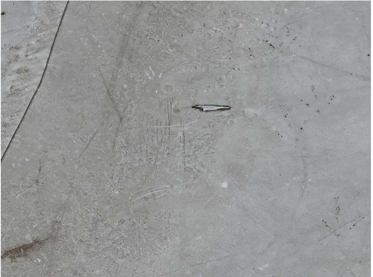
73 73-Mechanical Damage Date Taken: 4/21/2025 Taken By: Angela Night Splits are present on the roof that potentially were caused by irregular handling by roof repair companies.
