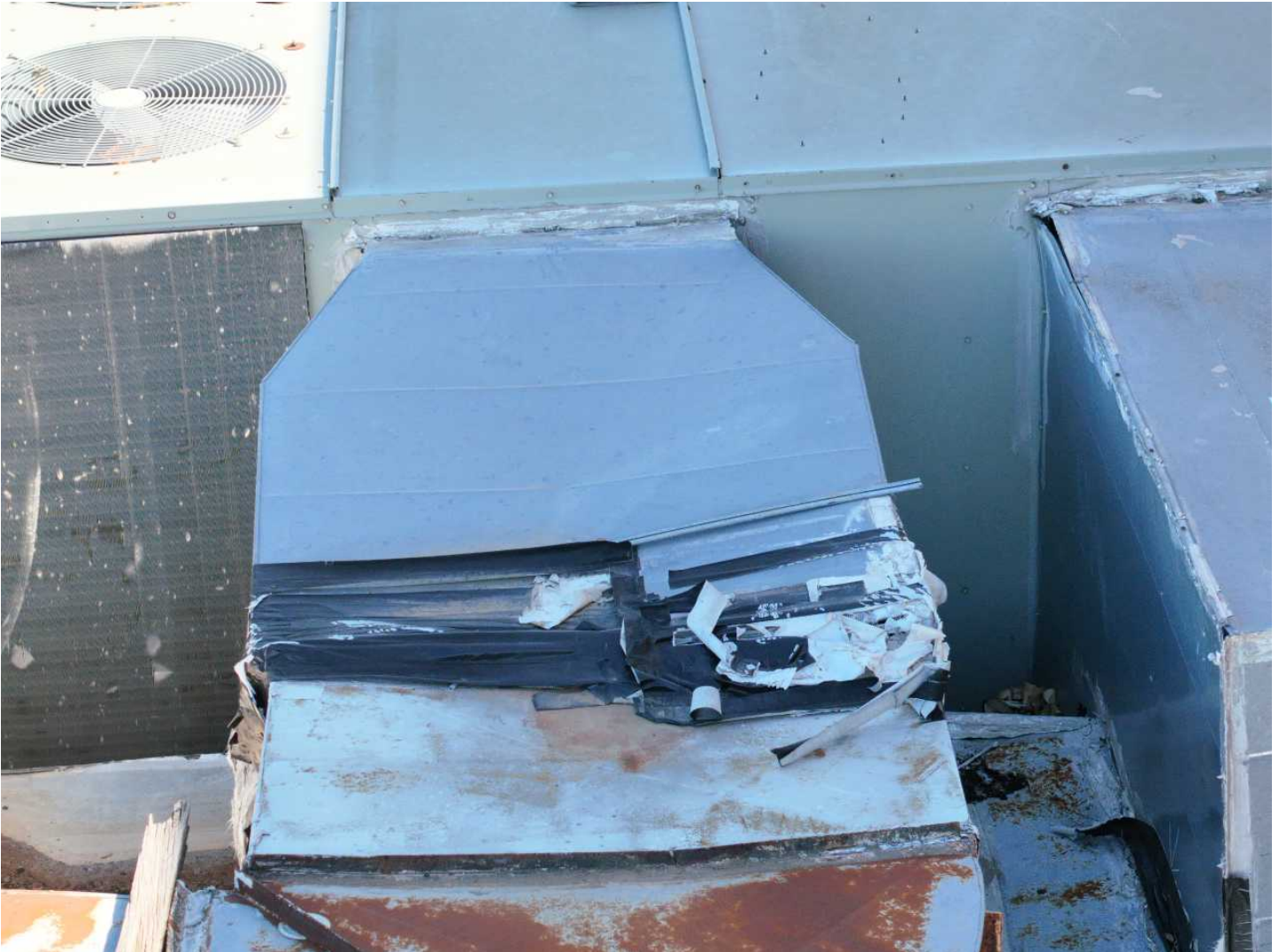
82 107-HVAC (Rectangular Duct) Date Taken: 4/21/2025 Taken By: Angela Night Exposed areas around the mechanical ducts were found atop the roof.
