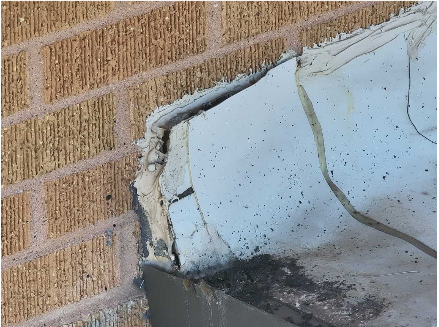
115 115-Failed Flashing Date Taken: 4/21/2025 Taken By: Angela Night Inadequate craftsmanship and unorganized placement indicative of a poor repair job or uncertified contractor.
