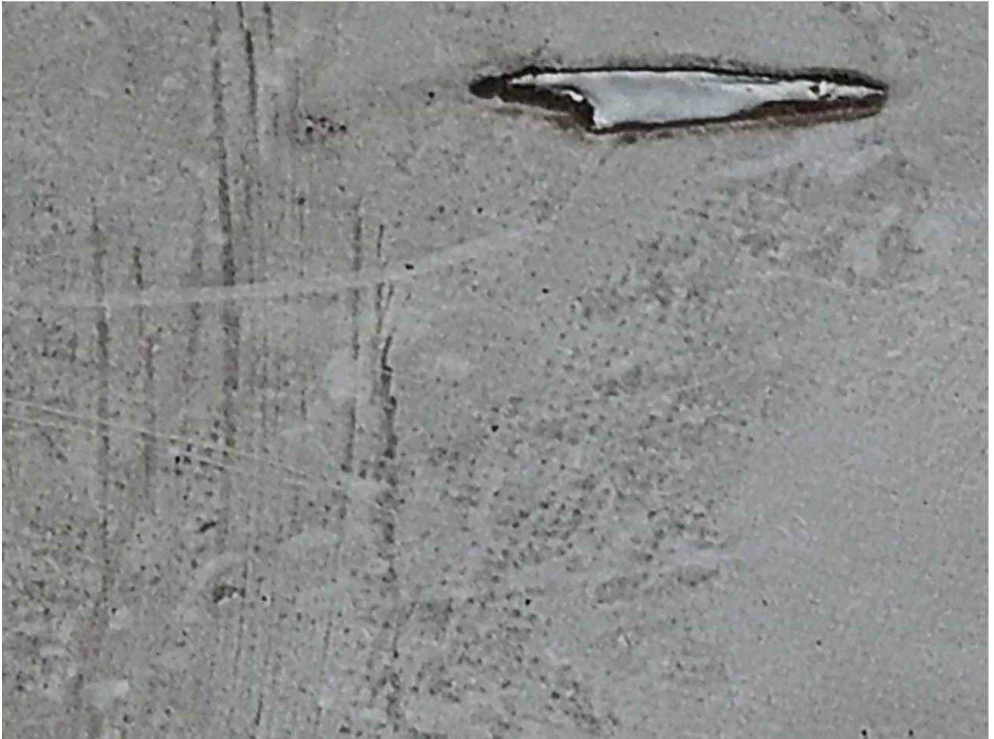
71 71-Mechanical Damage Date Taken: 4/21/2025 Taken By: Angela Night Splits are present on the roof that potentially were caused by irregular handling by roof repair companies.
