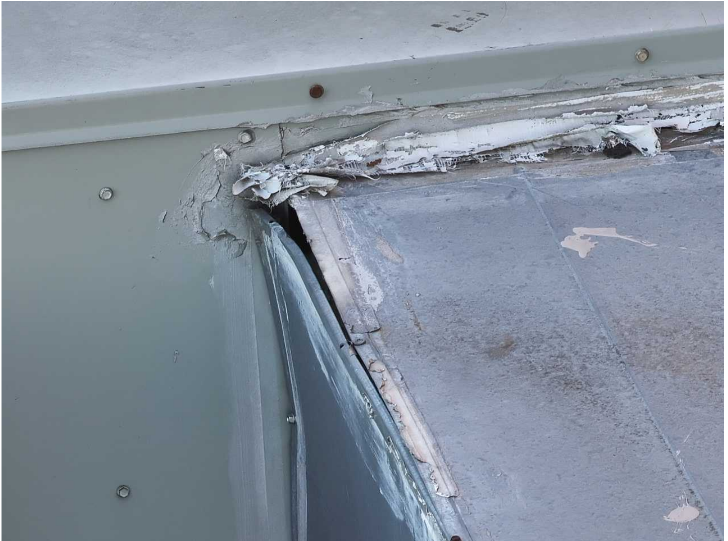
80 109-HVAC (Rectangular Duct) Date Taken: 4/21/2025 Taken By: Angela Night Exposed areas around the mechanical ducts were found atop the roof.
