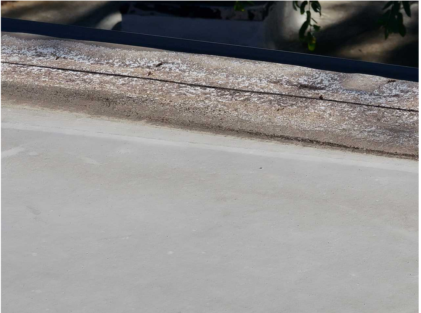
107 102-Loose Seams Date Taken: 4/21/2025 Taken By: Angela Night Edges around the roof membrane are separating from their seams due to poor installation and gap movement.
