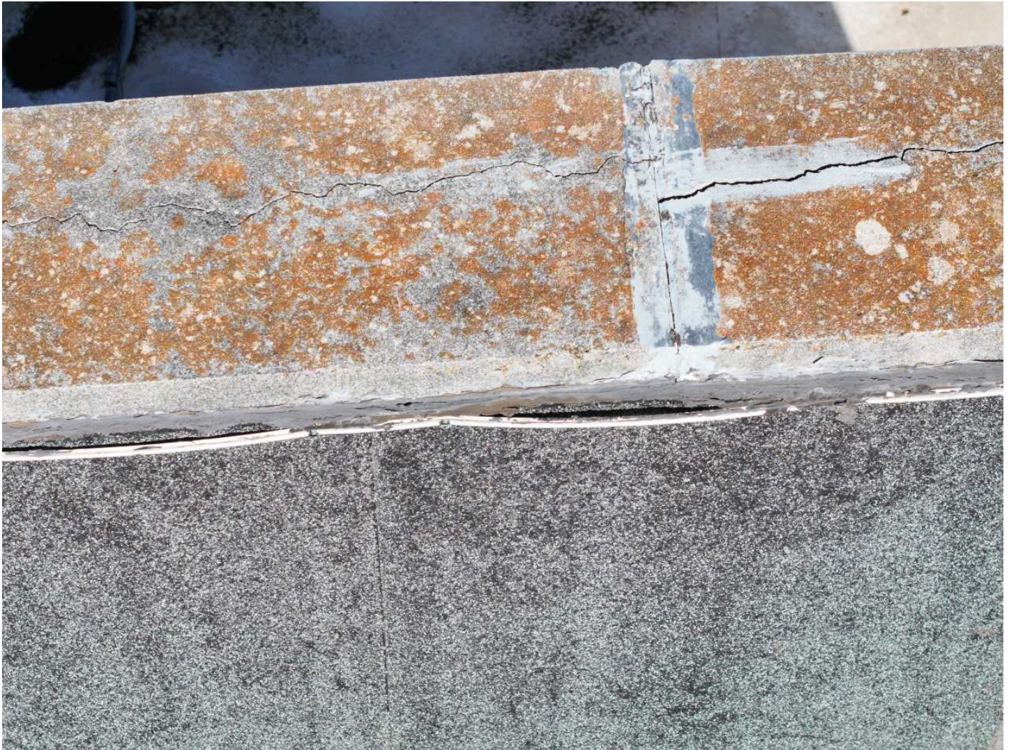
96 91-Loose Seams Date Taken: 4/21/2025 Taken By: Angela Night Edges around the roof membrane are separating from their seams due to poor installation and gap movement.
