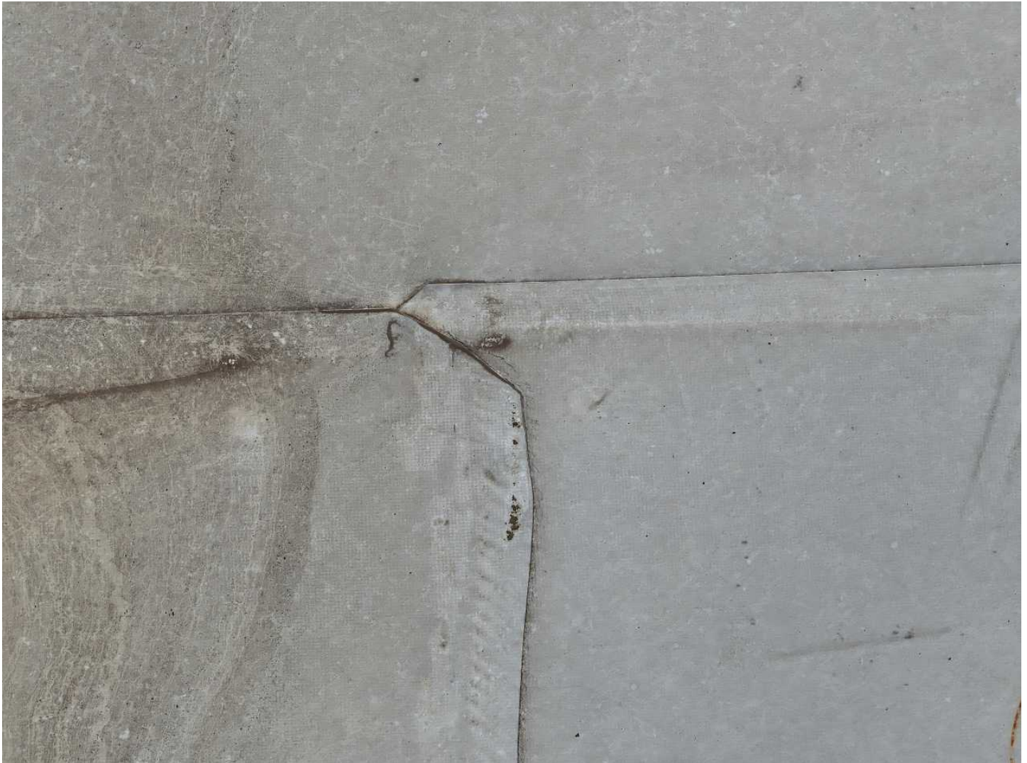
109 104-Loose Seams Date Taken: 4/21/2025 Taken By: Angela Night Edges around the roof membrane are separating from their seams due to poor installation and gap movement.
