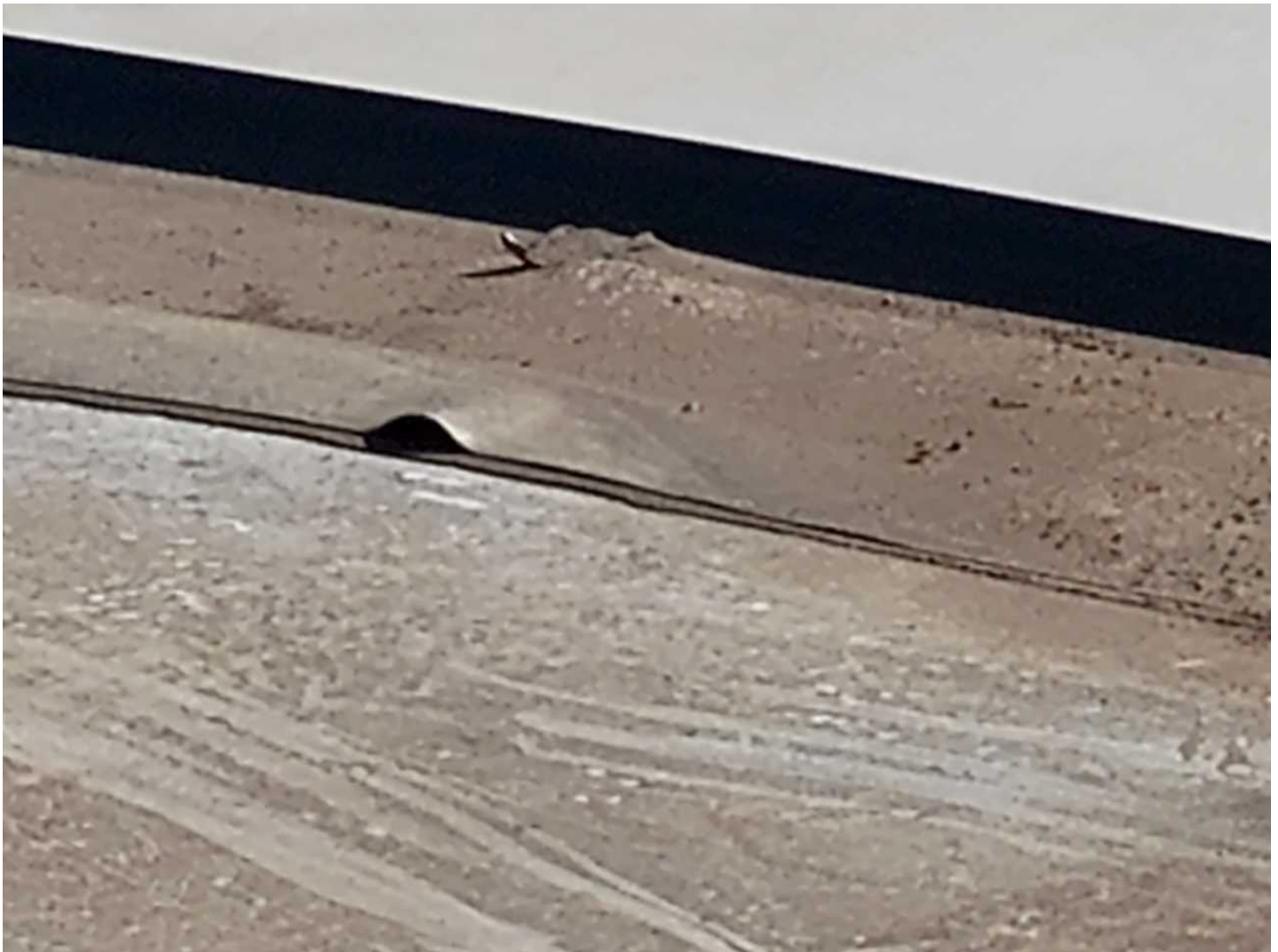
102 97-Loose Seams Date Taken: 4/21/2025 Taken By: Angela Night Edges around the roof membrane are separating from their seams due to poor installation and gap movement.
