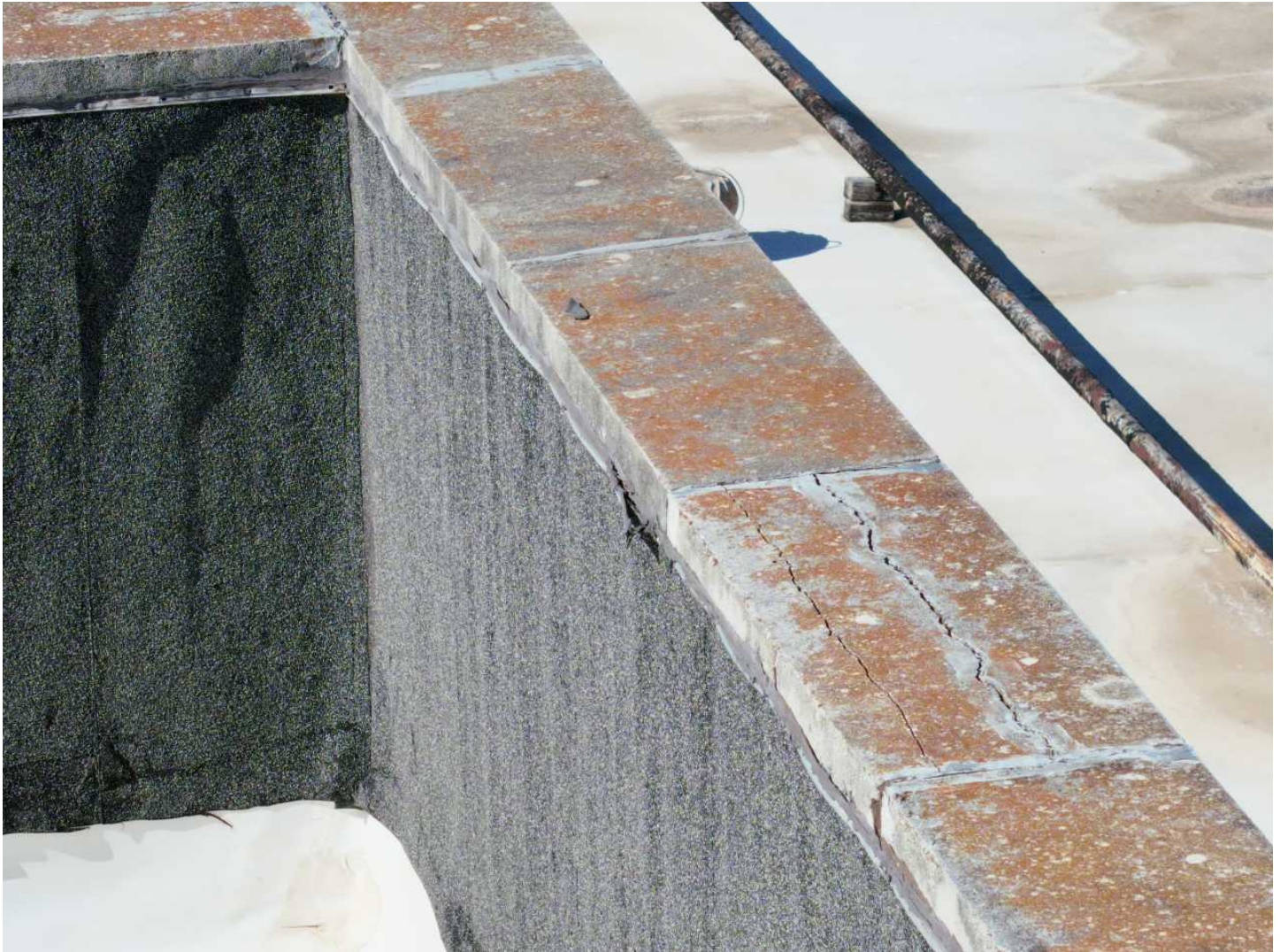
92 87-Loose Seams Date Taken: 4/21/2025 Taken By: Angela Night Edges around the roof membrane are separating from their seams due to poor installation and gap movement.
