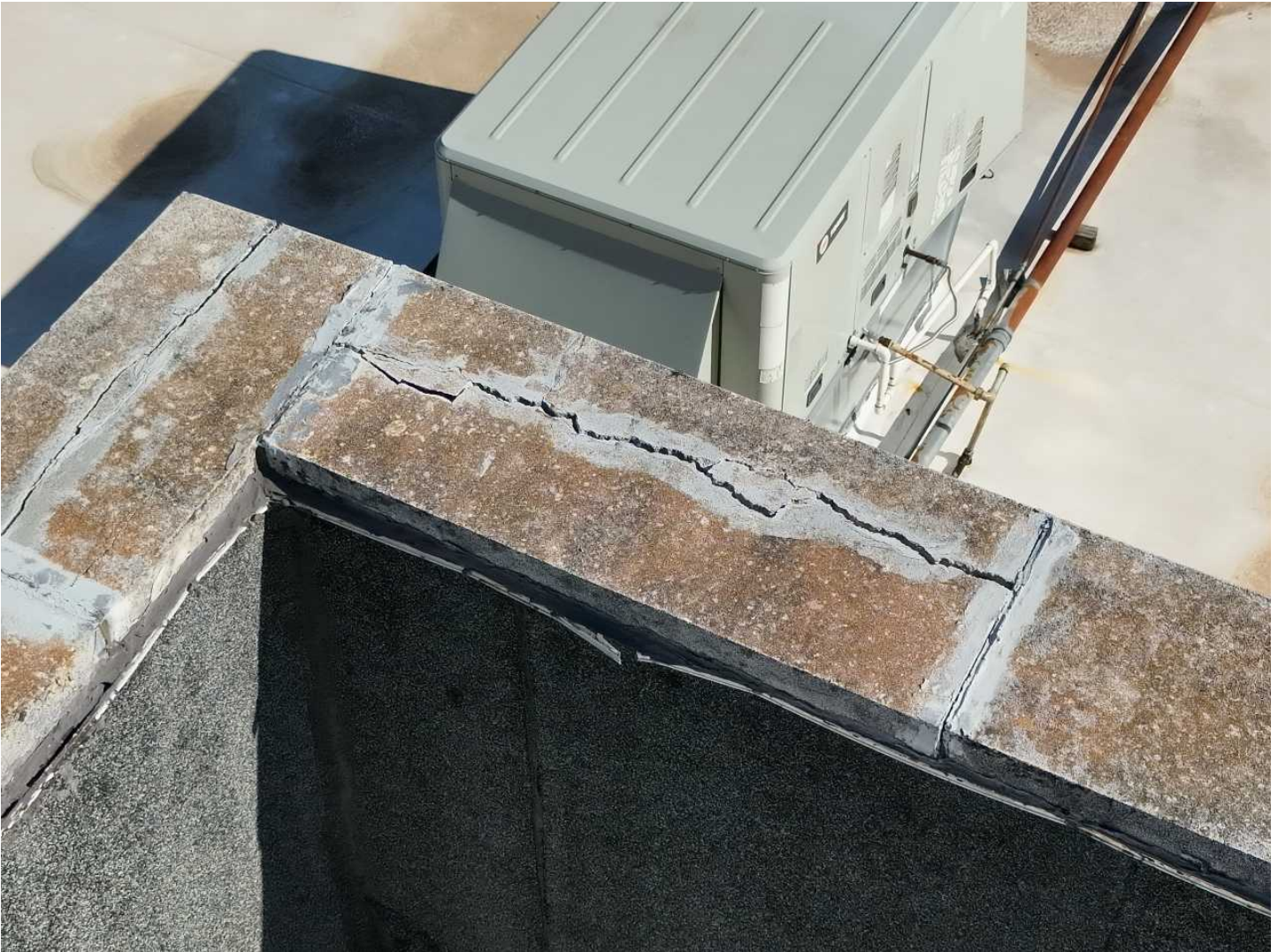
98 93-Loose Seams Date Taken: 4/21/2025 Taken By: Angela Night Edges around the roof membrane are separating from their seams due to poor installation and gap movement.
