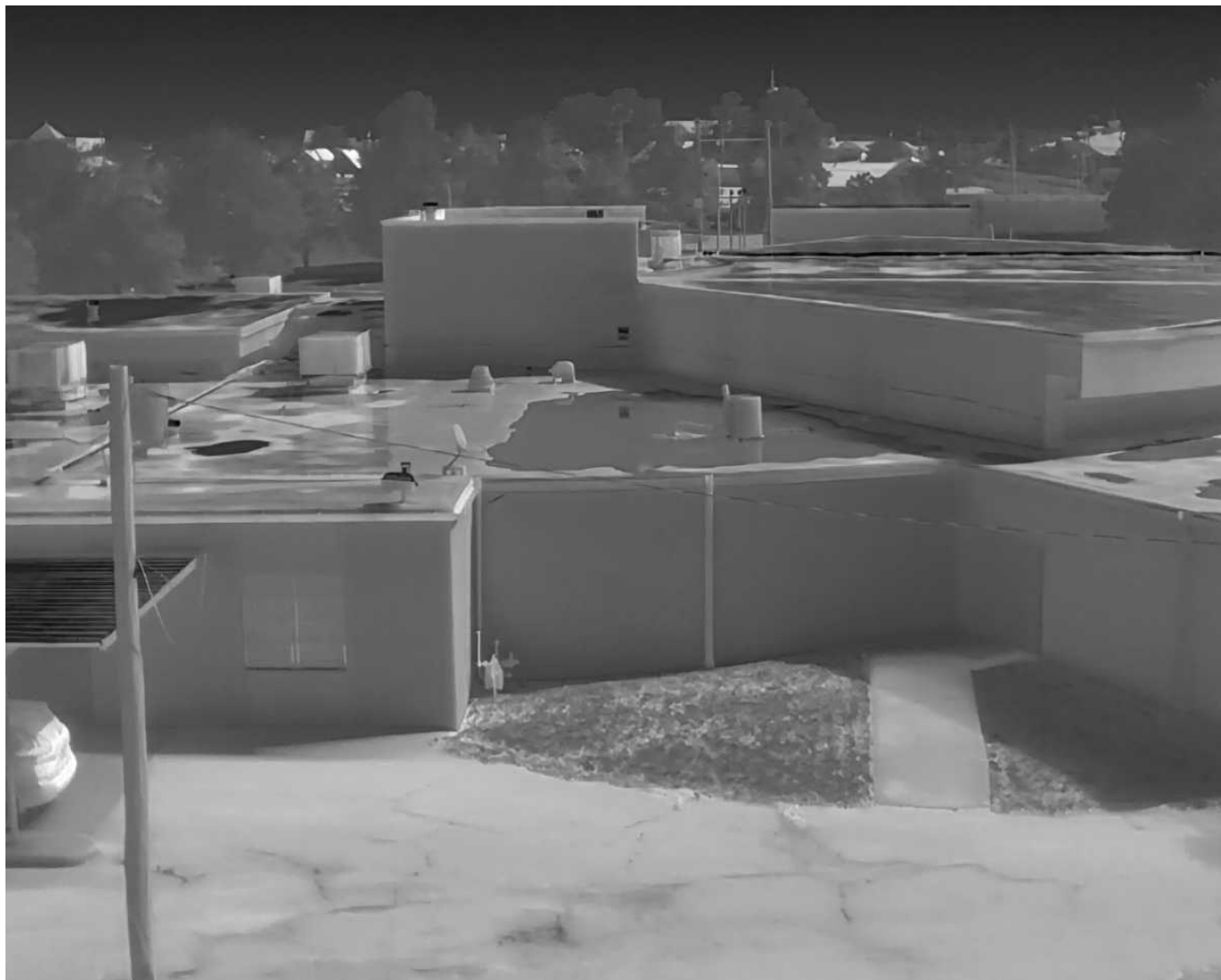
5 5-Ponding Date Taken: 4/21/2025 Taken By: Angela Night IR photos were taken in this instance to reflect the ponding of water due to leveling issues.
