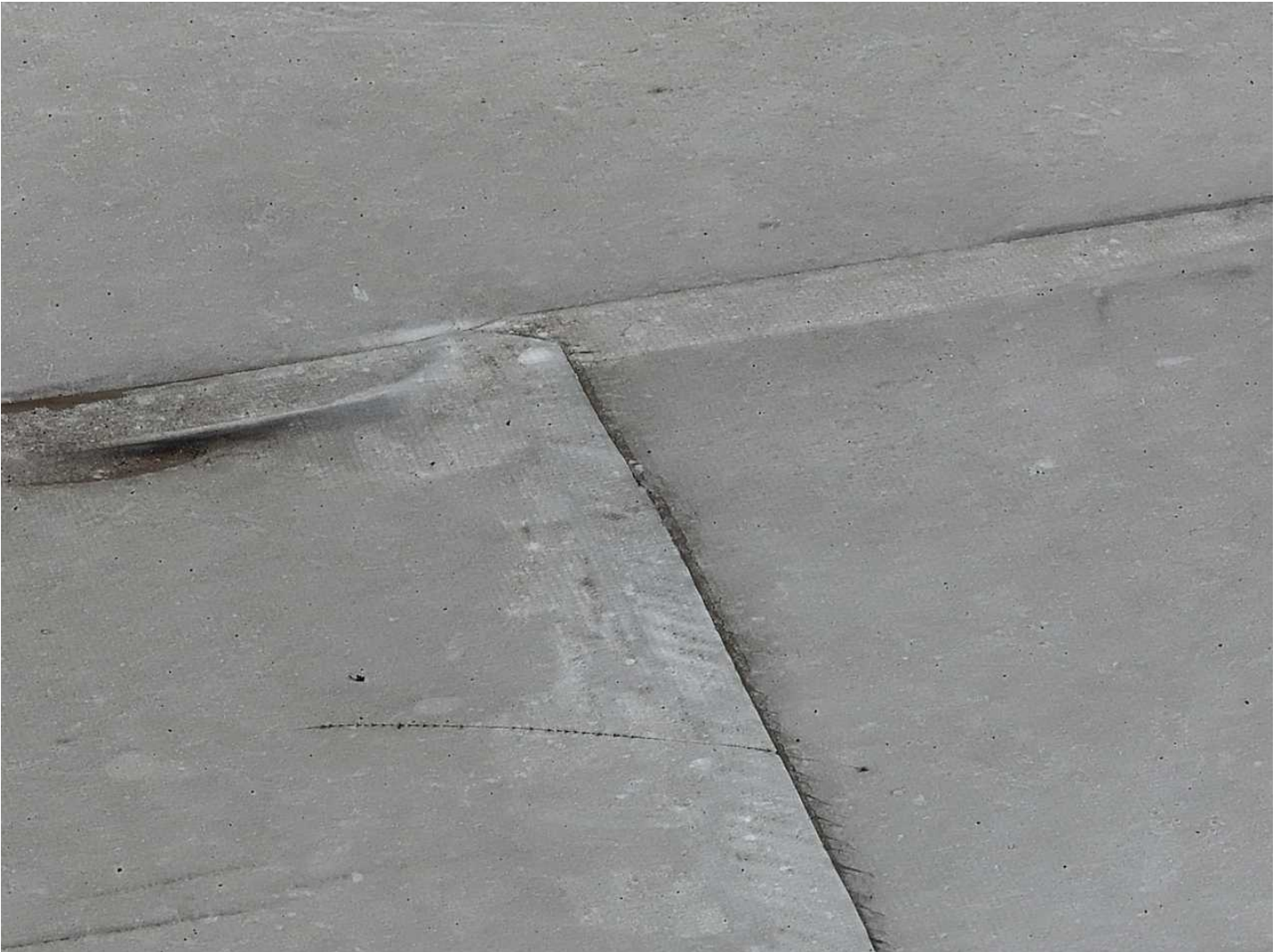
108 103-Loose Seams Date Taken: 4/21/2025 Taken By: Angela Night Edges around the roof membrane are separating from their seams due to poor installation and gap movement.
