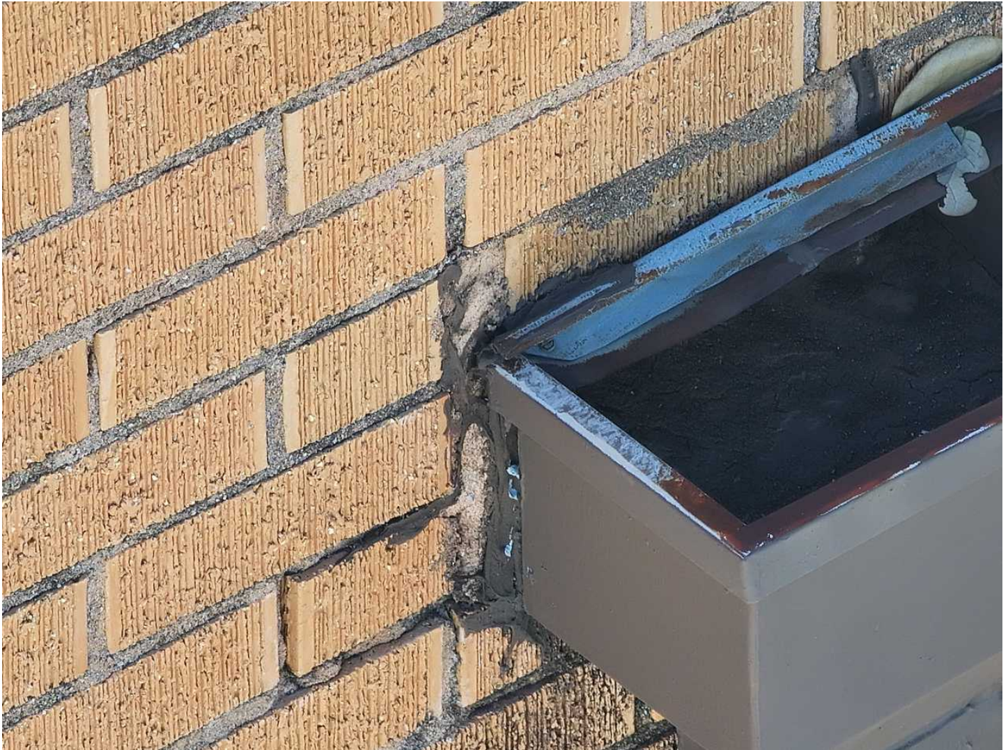
122 122-Conductor Head Need scrapped around and resealed
