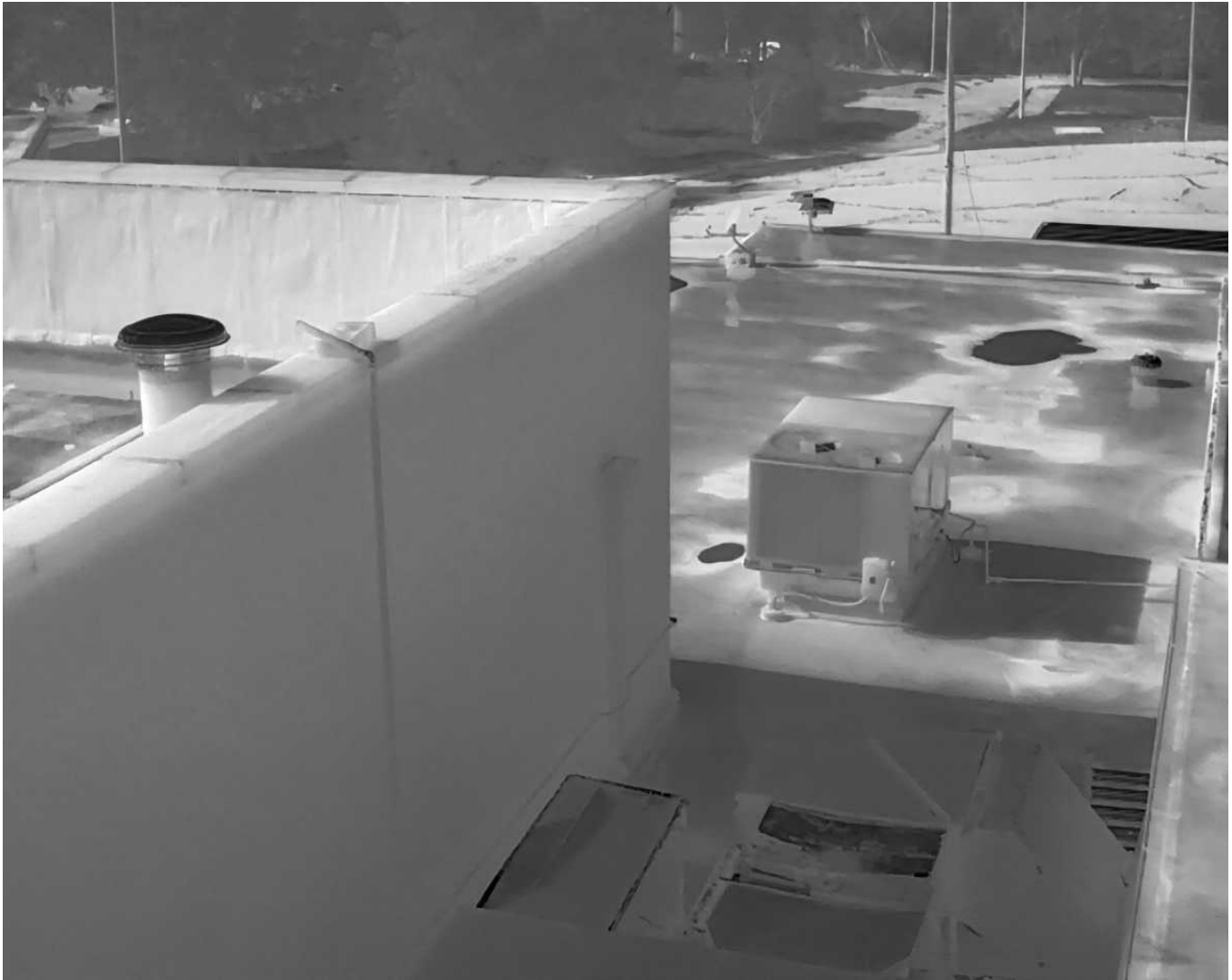
99 94-Loose Seams Date Taken: 4/21/2025 Taken By: Angela Night Edges around the roof membrane are separating from their seams due to poor installation and gap movement.
