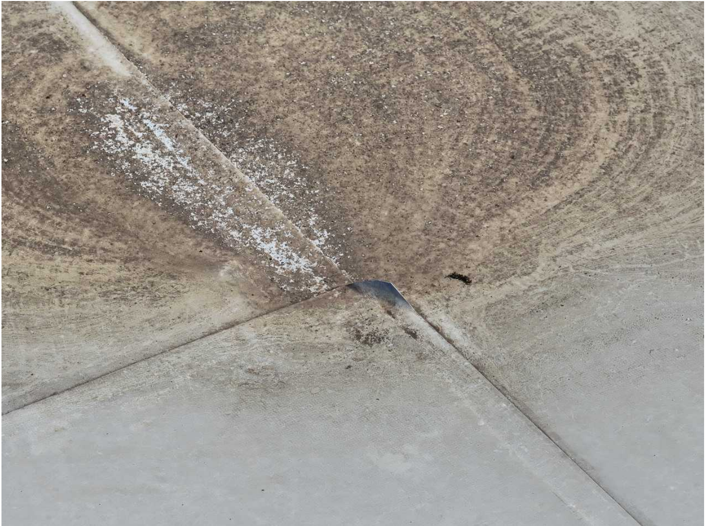
110 105-Loose Seams Date Taken: 4/21/2025 Taken By: Angela Night Edges around the roof membrane are separating from their seams due to poor installation and gap movement.
