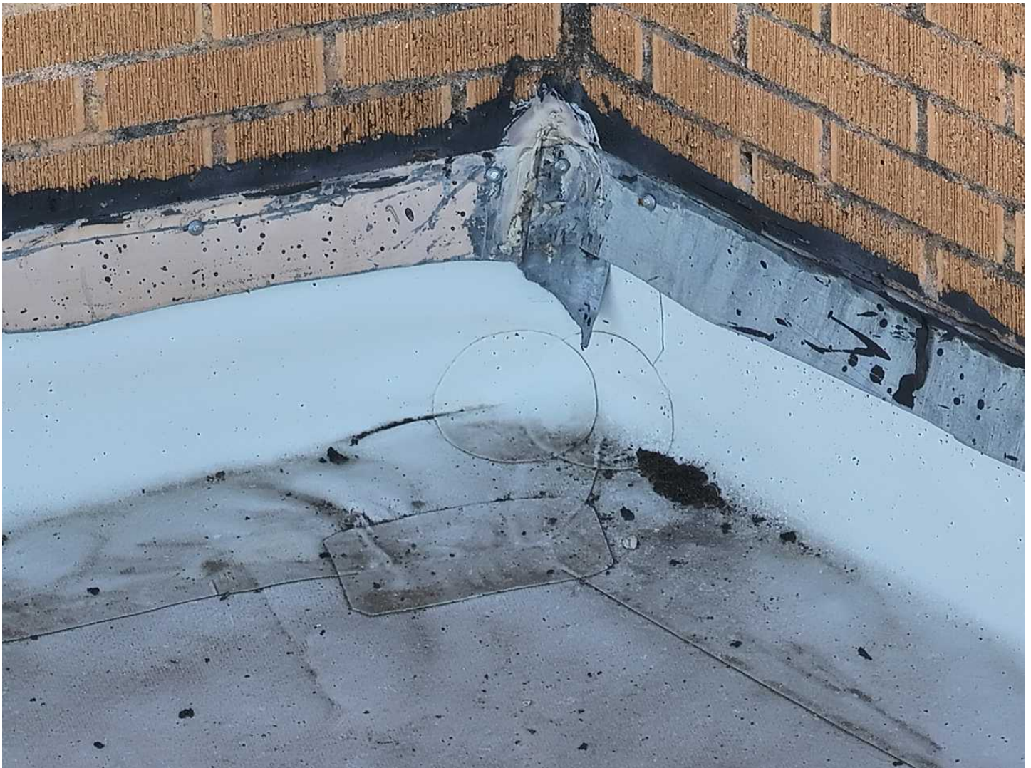
111 111-Failed Flashing Date Taken: 4/21/2025 Taken By: Angela Night Inadequate craftsmanship and unorganized placement indicative of a poor repair job or uncertified contractor.
