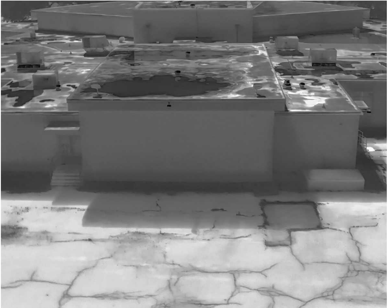
3 3-Ponding Date Taken: 4/21/2025 Taken By: Angela Night IR photos were taken in this instance to reflect the ponding of water due to leveling issues.
