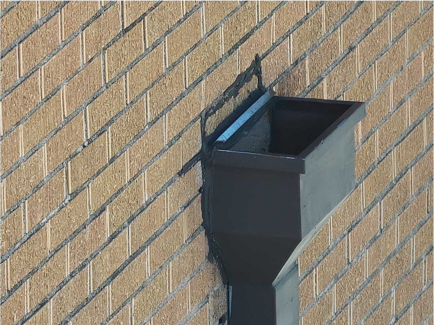
126 126-Conductor Head Need scrapped around and resealed
