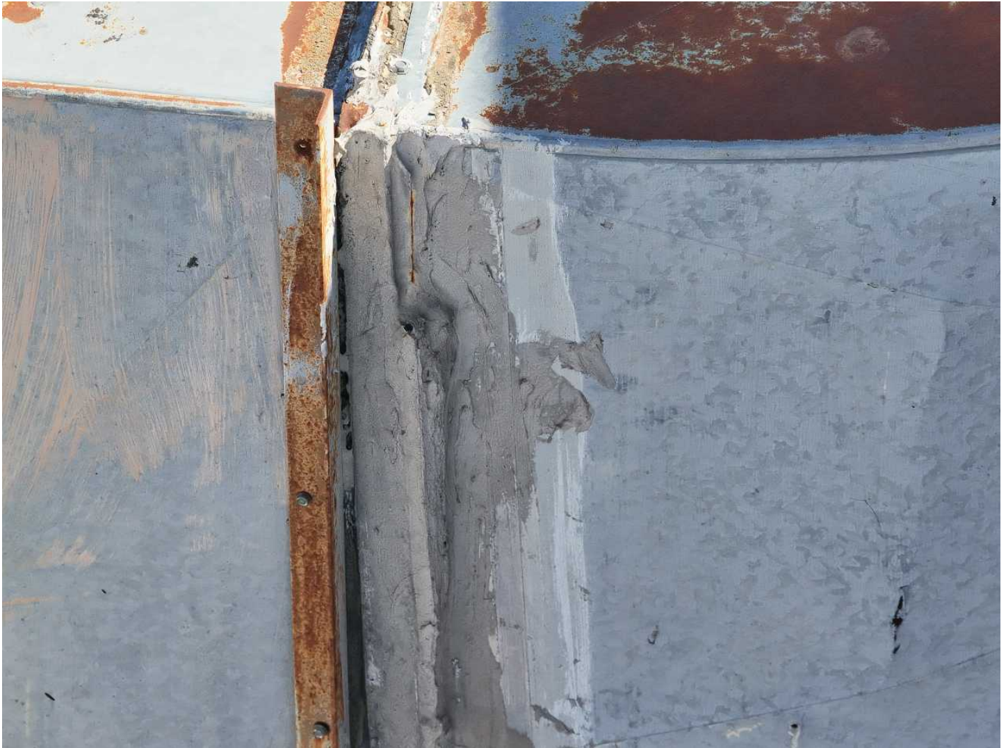
83 106-HVAC (Rectangular Duct) Date Taken: 4/21/2025 Exposed areas around the mechanical ducts were found atop the roof.
