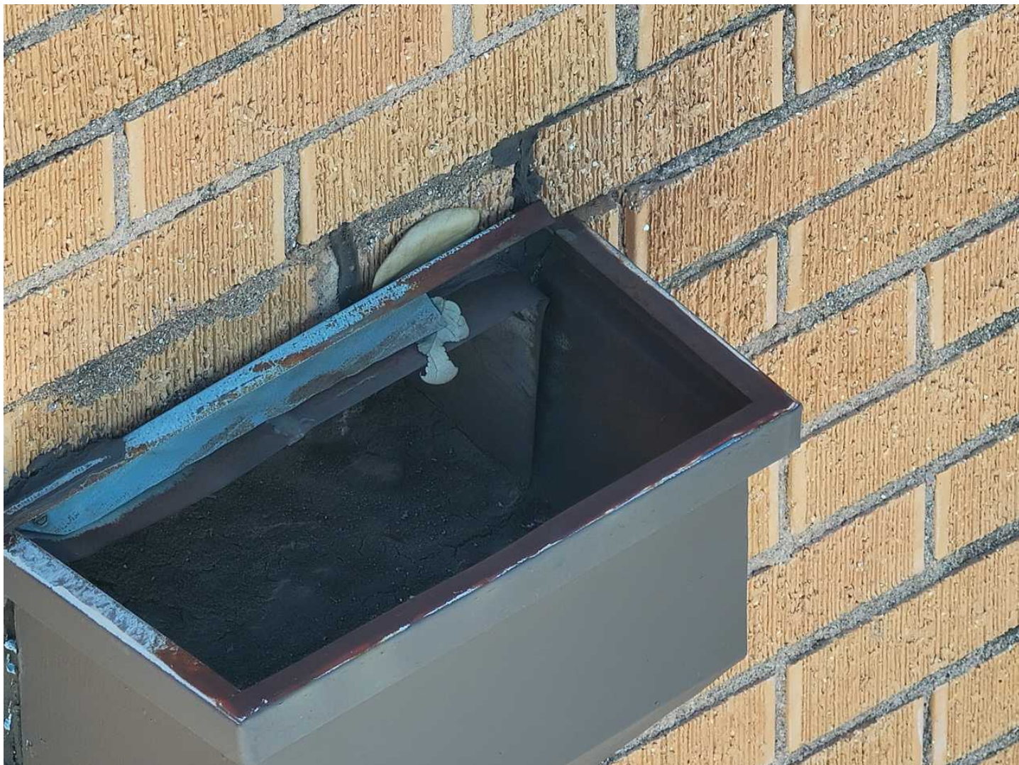
123 123-Conductor Head Need scrapped around and resealed
