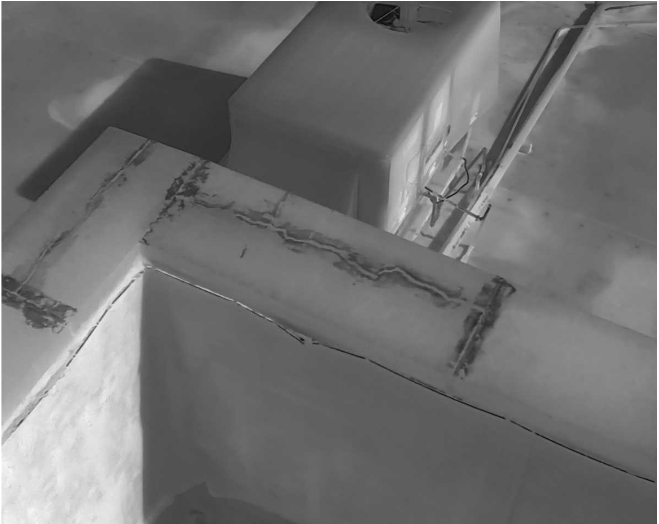
97 92-Loose Seams Date Taken: 4/21/2025 Taken By: Angela Night Edges around the roof membrane are separating from their seams due to poor installation and gap movement.
