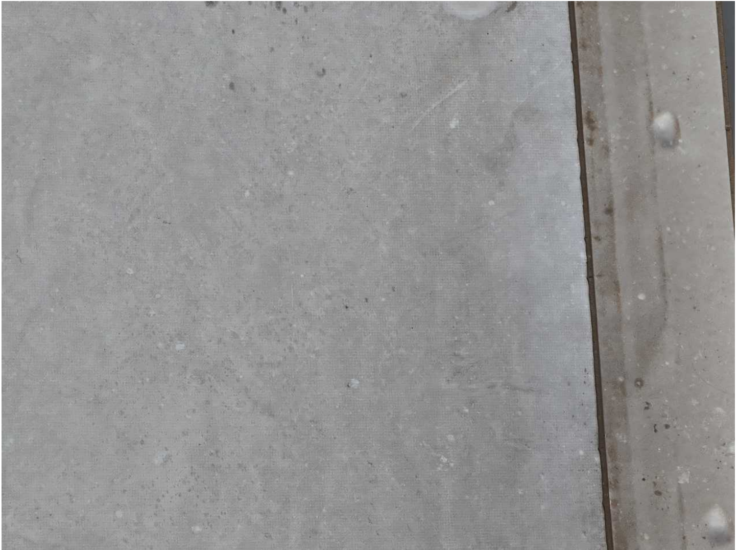
61 61-Indicative Hail Date Taken: 4/21/2025 Taken By: Angela Night Natural power wash markings from hail that was present (non damaging).
