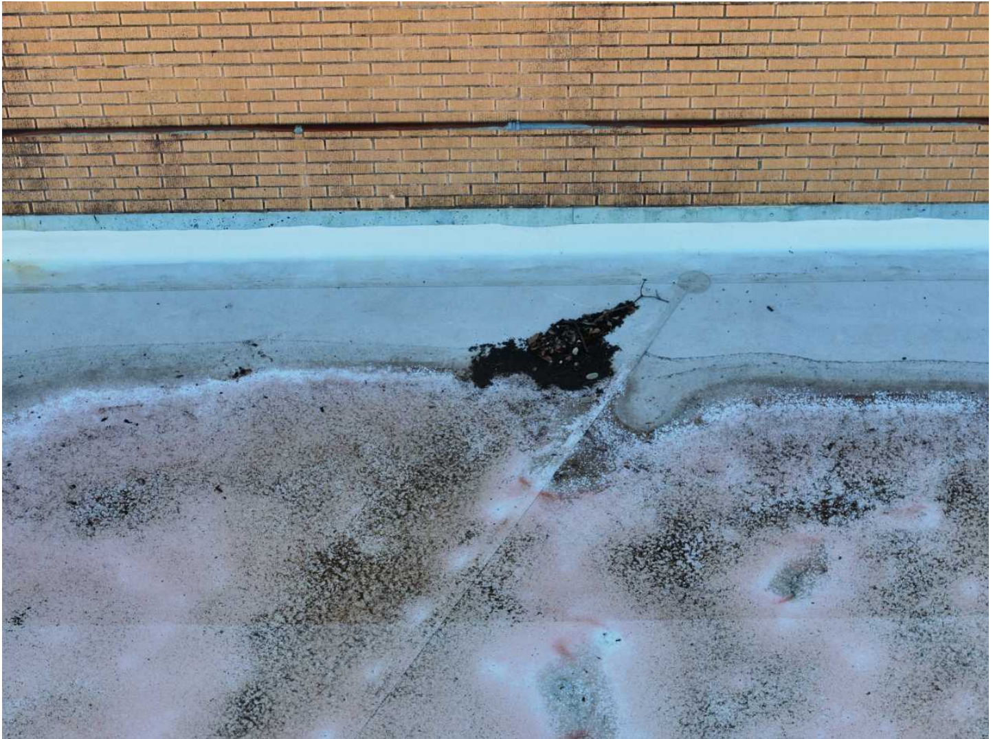
112 112-Failed Flashing Date Taken: 4/21/2025 Taken By: Angela Night Inadequate craftsmanship and unorganized placement indicative of a poor repair job or uncertified contractor.
