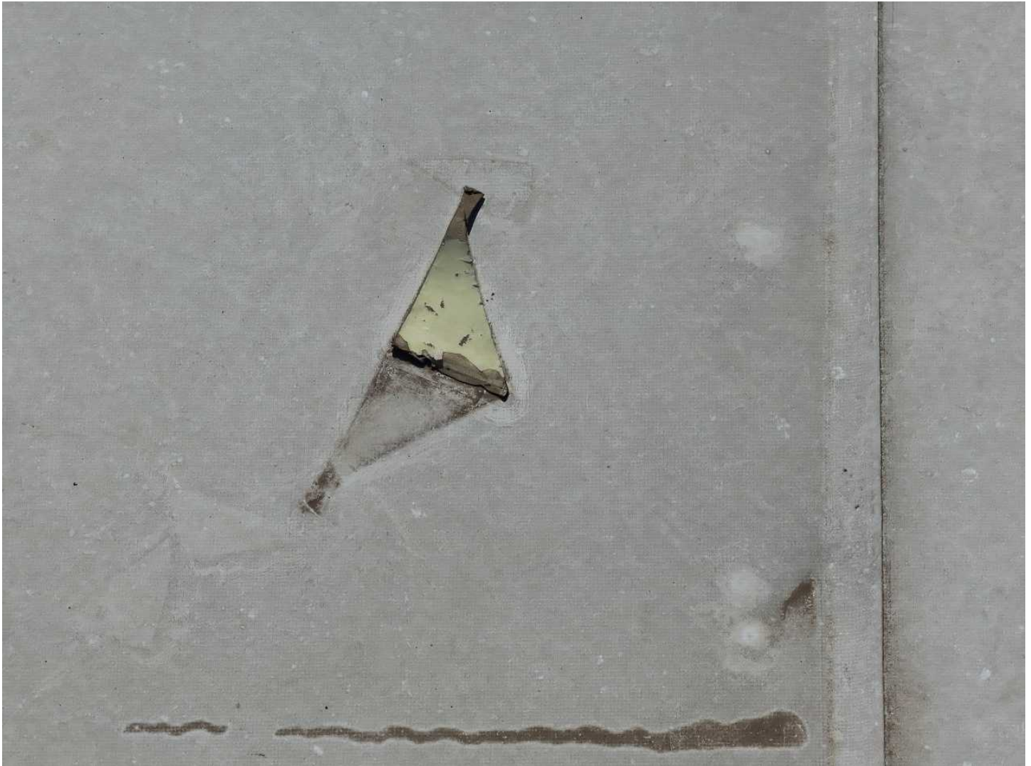
76 76-Mechanical Damage Date Taken: 4/21/2025 Taken By: Angela Night Splits are present on the roof that potentially were caused by irregular handling by roof repair companies.
