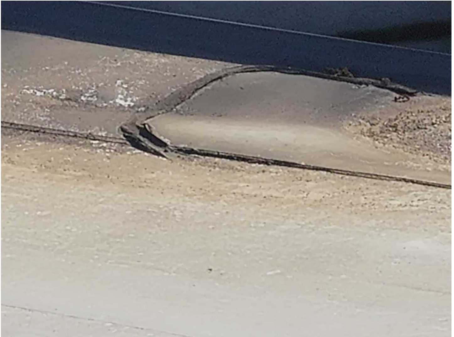
106 101-Loose Seams Date Taken: 4/21/2025 Taken By: Angela Night Edges around the roof membrane are separating from their seams due to poor installation and gap movement.
