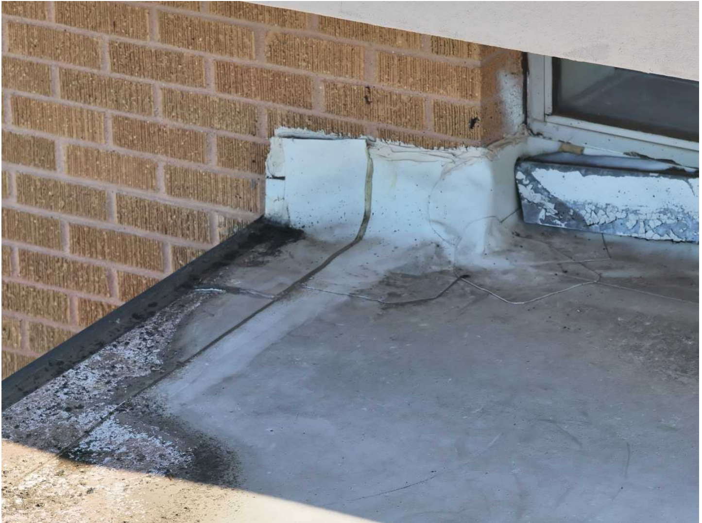
116 116-Failed Flashing Date Taken: 4/21/2025 Taken By: Angela Night Inadequate craftsmanship and unorganized placement indicative of a poor repair job or uncertified contractor.
