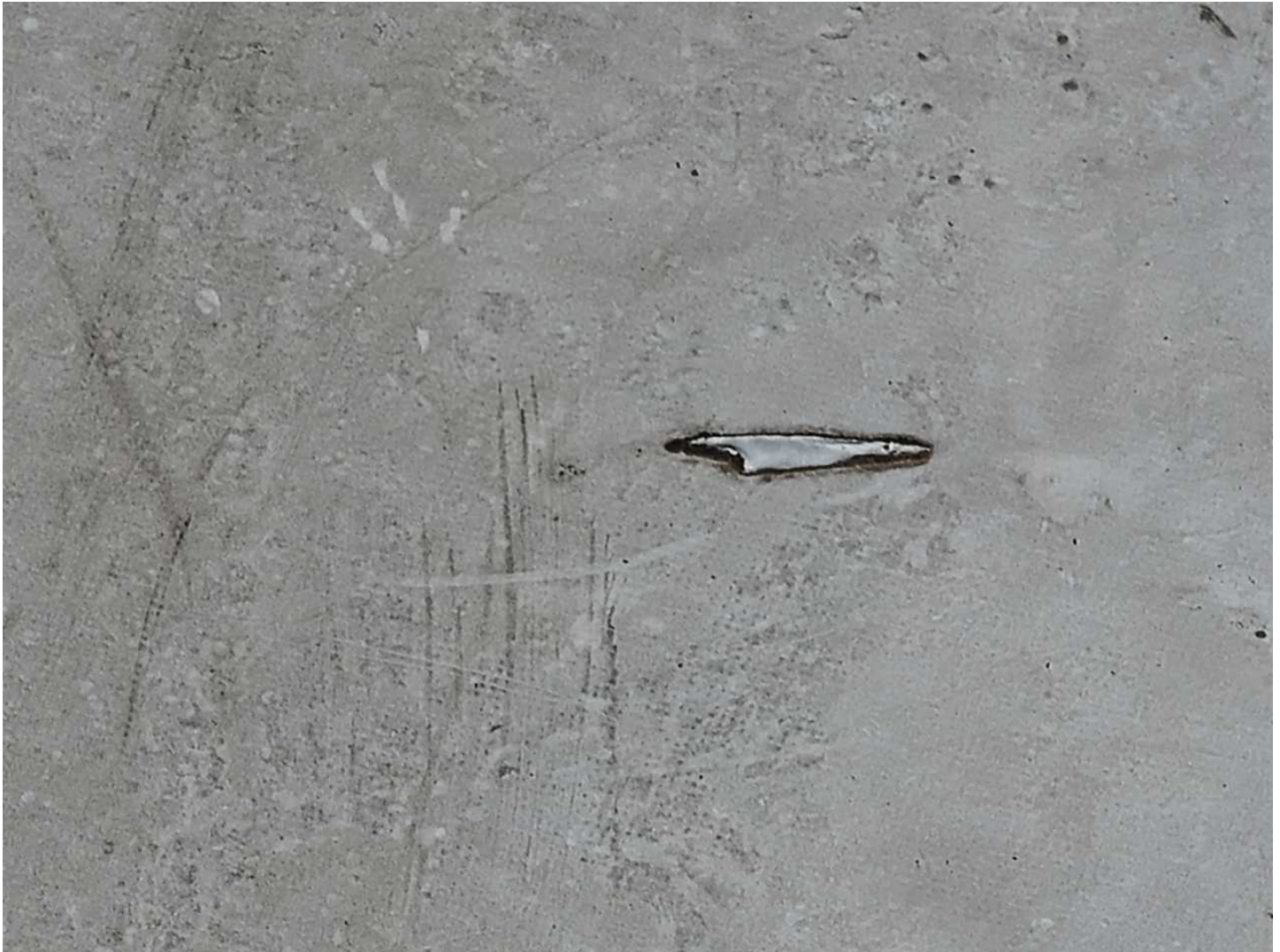
72 72-Mechanical Damage Date Taken: 4/21/2025 Taken By: Angela Night Splits are present on the roof that potentially were caused by irregular handling by roof repair companies.
