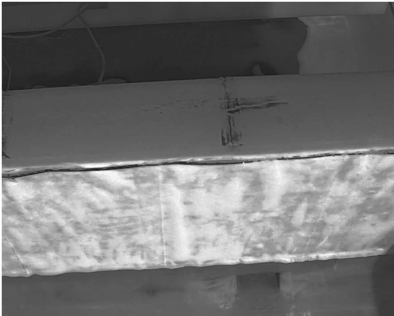
94 89-Loose Seams Date Taken: 4/21/2025 Taken By: Angela Night Edges around the roof membrane are separating from their seams due to poor installation and gap movement.
