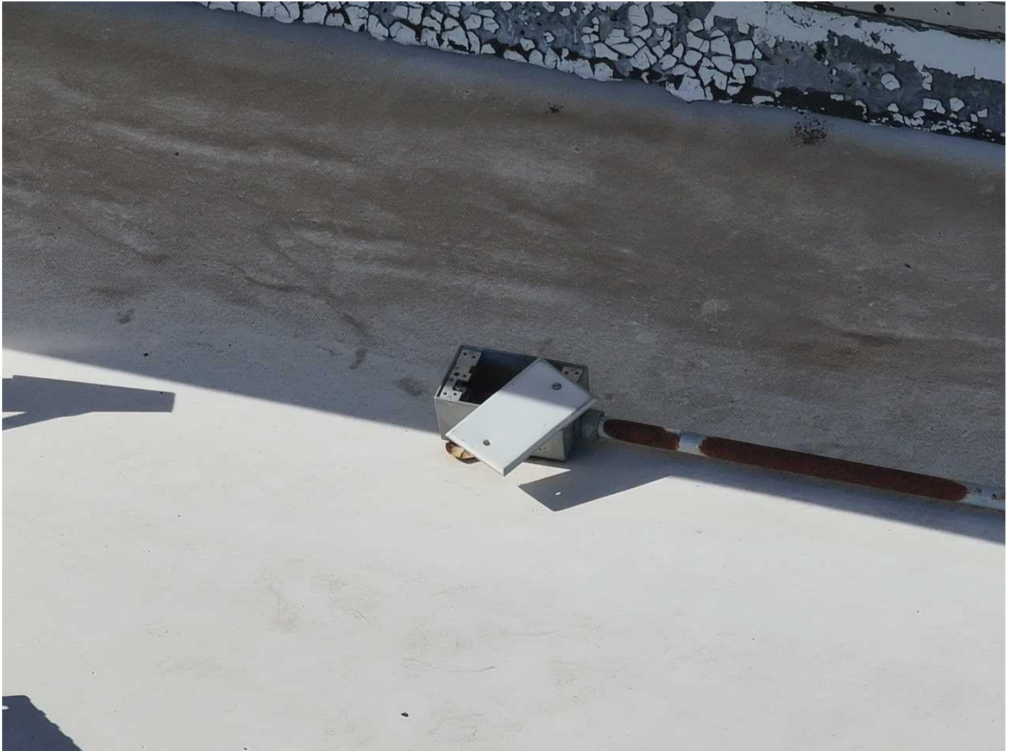
127 127-Misc Date Taken: 4/21/2025 Taken By: Angela Night All unused fixtures, whether electrical or mechanical need not be left on the roof. A crowded roof can result in assessment delays, improper weight distribution and become a safety hazard.
