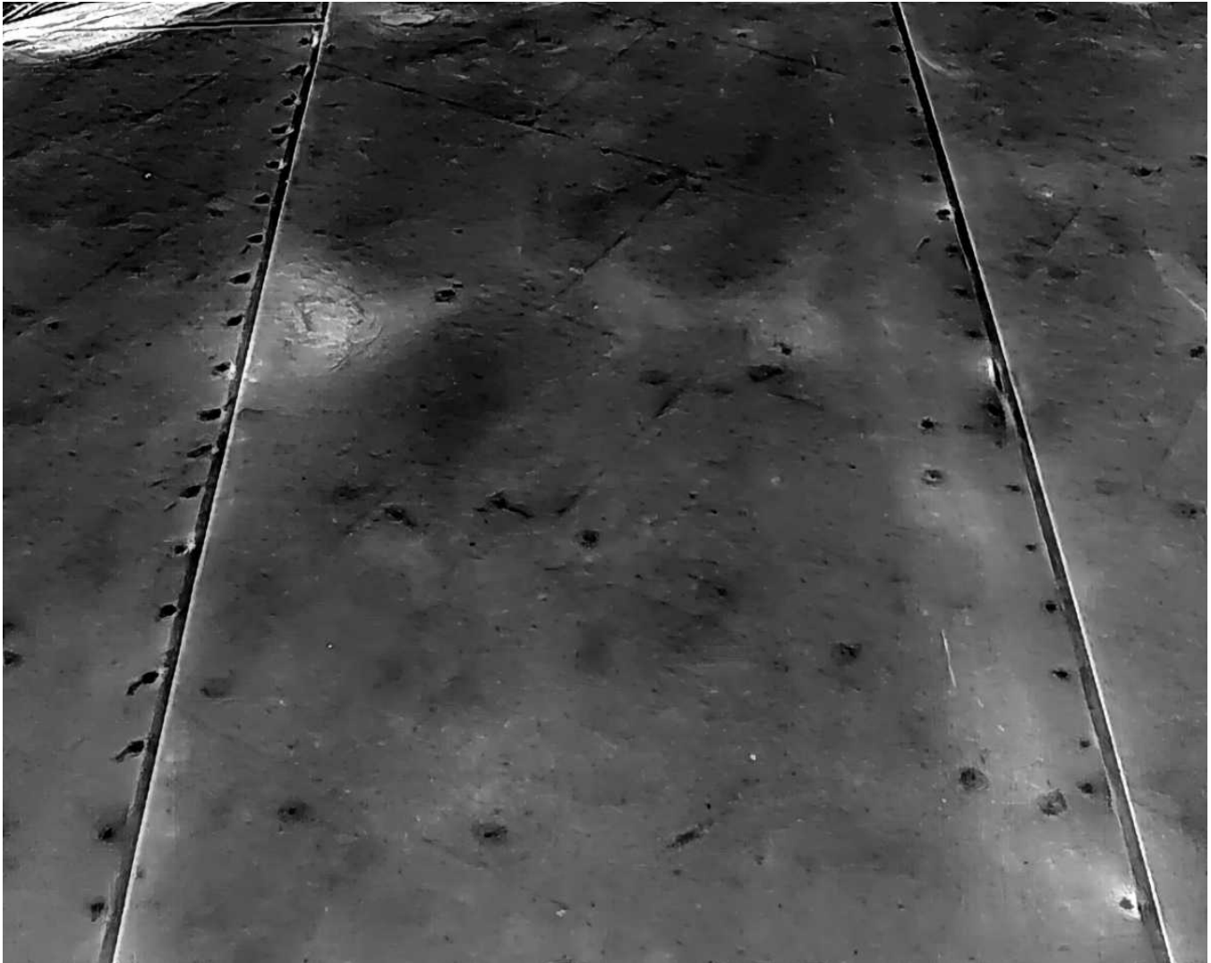
100 95-Loose Seams Date Taken: 4/21/2025 Taken By: Angela Night Edges around the roof membrane are separating from their seams due to poor installation and gap movement.
