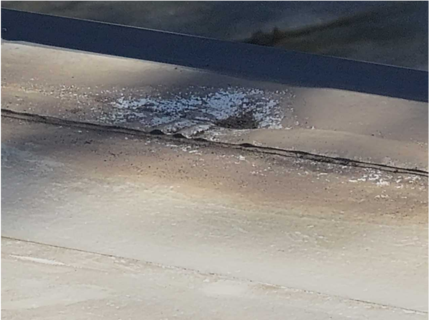
104 99-Loose Seams Date Taken: 4/21/2025 Taken By: Angela Night Edges around the roof membrane are separating from their seams due to poor installation and gap movement.
