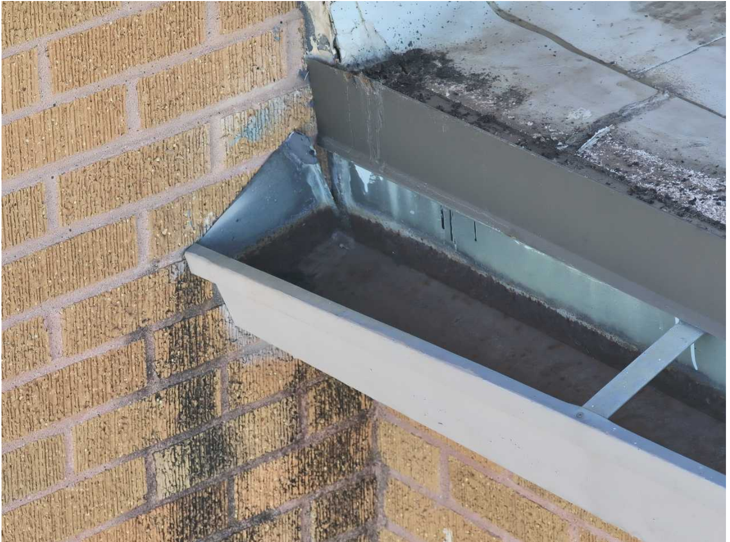
114 114-Failed Flashing Date Taken: 4/21/2025 Taken By: Angela Night Inadequate craftsmanship and unorganized placement indicative of a poor repair job or uncertified contractor.
